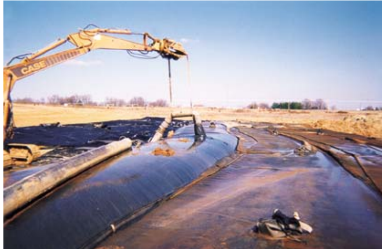
Photo 3: Tube being filled with dredged material.
