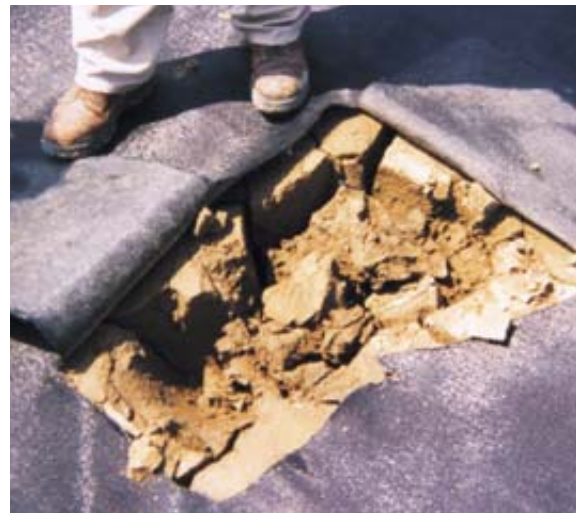
Photo 4: Cutaway section of tube showing material once it has been dewatered.
