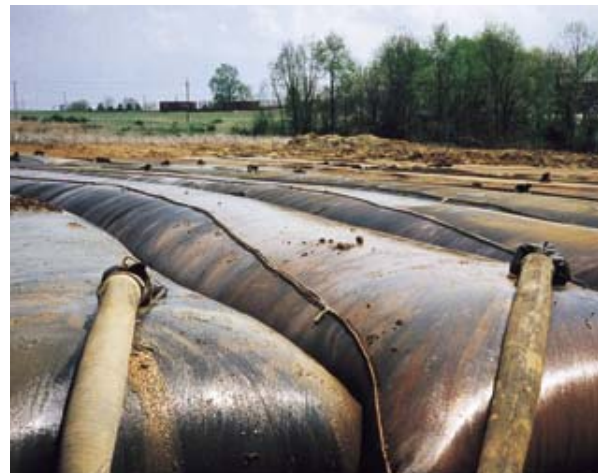
Photo 2: The dredged material was pumped into several 200-foot-long geotextile tubes.
