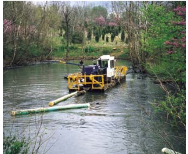
Photo 1: Dredging to remove organic sediment.
