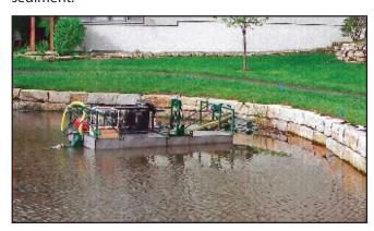
The sediment was pumped from pond 2 into a geotextile 4x6 45 ft. circumference x 25 ft. long Envirotube placed in a cul de sac 300 feet from the pond. Pallets and firewood was used to stabilize the tube to prevent rolling.
