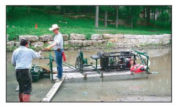
Pond 2 had silted in with three to four feet of organic, clay and gritty sediment. There were also some stones and trash.
